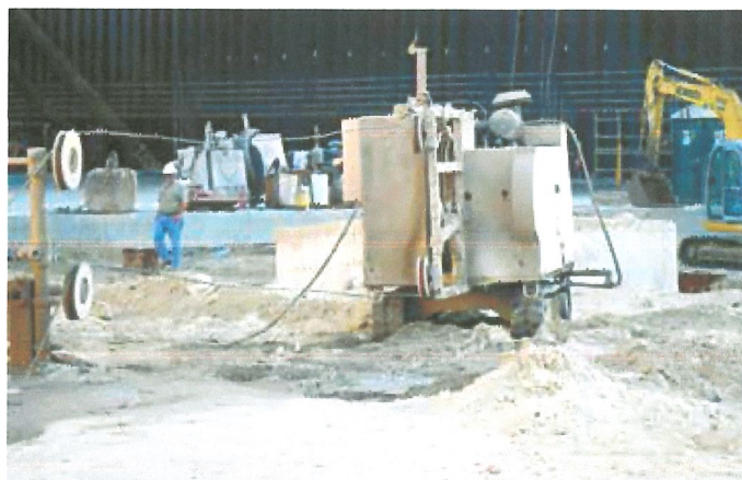
Wire saw units from several locations across the U.S. were brought to the dock.
