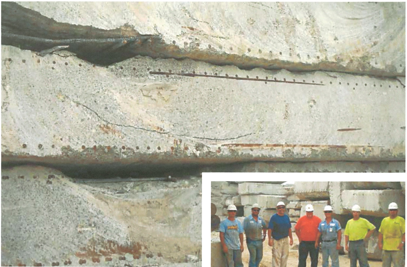
Operators cut approximately 44,700 cubic feet of concrete.
