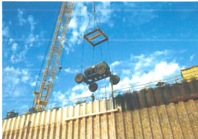
Tools and equipment were lowered to the dock basin by crane.
